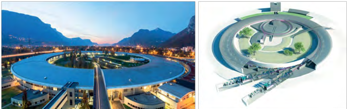
FIGURE 9 The European Synchrotron Radiation Facility (ESRF) in Grenoble has recently begun operating the new "Extremely Brilliant Source," the first fourth-generation high-energy synchrotron. In this configuration, high-energy electrons are accelerated within the circular tunnel of the synchrotron ring. The subsequent emission of X-rays is then utilised for diagnostic purposes. © Courtesy of European Synchrotron Radiation Facility, ESRF, Grenoble.
